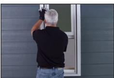
Apply flashing tape to the window sill, butting it up to the interior stop. Flashing tape should measure the same width of the window frame and the depth of the replacement window frame. Use the J-roller to remove any air pockets.
