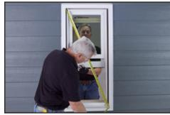
**8** Apply OSI® QUAD® foam into the gap between the pocket window and the framing at the head and side jambs. Do not apply foam between the pocket window sill and the window sill.
