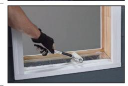
**5 Apply a bead of OSI® QUAD® Max** between the sill flashing and the side jamb on both sides.
