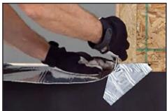
Make relief cuts in the corners and then fold the flashing tape onto the apron. Use the J-roller to remove any air pockets.
