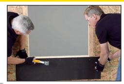
Measure the depth of the window frame, but do not include the extension jamb if present. Add a 1/4", measure that total on the rough opening sill, and mark it with a pencil. This will show you where the interior edge of the flashing should be.
