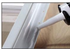
Apply a discontinuous bead on the bottom flange. Leaving a minimum of a 2" gap at each corner and every 6" to 8".
