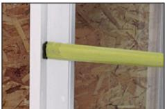
**Apply corner guards** at sill and side jamb joints by using a 6" x 6" piece of flashing tape, cutting it into a "butterfly" shape and forming into the corners.
