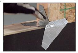
Cut the sill flashing to the width of the rough opening plus 12". Align the flashing tape with the pencil marks from step 2 and center the tape in the rough opening onto the sill and extend it up each side jamb 6".
