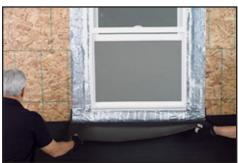
Seal the next layer of WRB to the flashing at the window sides and head jambs using either OSI® QUAD® Max sealant or WRB joint tape.
