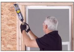
**Allow 25 to 35 minutes** for foam to cure and trim off the excess with a sharp knife.
