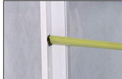
**Apply corner guards** at sill and side jamb joints by using a 6" x 6" piece of flashing tape, cutting it into a "butterfly" shape and forming into the corners.
