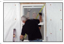
Install the window using all manufacturer's installation instructions and ensure the window operates properly. Tool any bulging sealant flat, so it doesn't interfere with future cladding installation.
