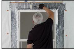
Pull down the top flap, and tape both 45-degree corners with flashing tape or WRB joint tape. Seal the WRB over the header with sealant or flashing tape.
