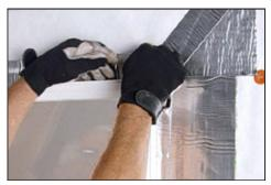
**From the interior** apply OSI® QUAD® foam into the gap between the window and the framing at the head, side and sill jambs. This must be a continuous seal with no visible shims.
