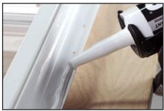
Apply a discontinuous bead on the bottom flange. Leaving a minimum of a 2" gap at each corner and every 6" to 8".
