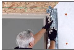
**Apply a second layer** of flashing tape to cover the window fin, buck edge and primary jamb overlapping at least 1". Use the J-roller to remove any air pockets.
