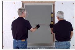
Install the window using all manufacturer's installation instructions and ensure the window operates properly. Tool any bulging sealant flat, so it doesn't interfere with future cladding installation.
