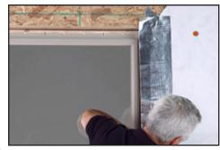
Make two relief cuts at the sill and head corners. Fold the remaining flashing tape into the opening over the primary jamb.
