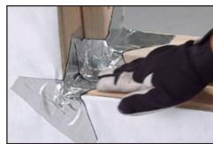
Cut the sill flashing to the width of the rough opening plus 12". Center the flashing tape on the exterior sill butting it to the exterior edge of the buck so that it extends up each side jamb 6".
