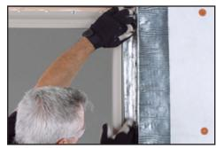
**Apply head flashing** with pre-cut relief cuts at the head and side jamb corners. Fold the remaining flashing into the opening over the primary head jamb and use the J-roller to remove any air pockets.
