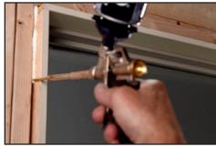
Allow 25 to 35 minutes for foam to cure and trim off the excess with a sharp knife.
