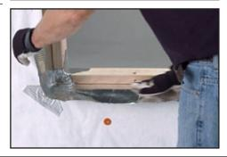
**Make relief cuts in the corners** and then fold the flashing tape onto the apron. Use the J-roller to remove any air pockets.
