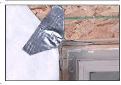
Measure and cut the side jamb flashing.
