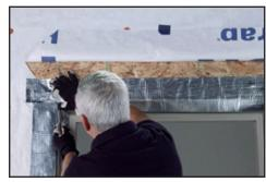
Apply a second layer of head flashing to cover the window fin, buck edge, and primary head flashing, overlapping the primary jamb flashing a minimum of 1". Use the J-roller to remove any air pockets.
