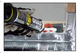
Apply a continuous 3/8" rounded bead of OSI® QUAD® Max to the head and side buck edges.
