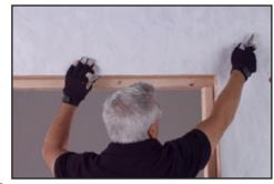
Measure the depth of the window frame, but do not include the extension jamb if present. Add a 1/4", measure that total on to the buck's rough sill, and mark it with a pencil. This will show you where the interior edge of the flashing should be.
