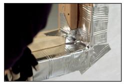
**Cut the sill flashing** to the width of the rough opening plus 12". Align the flashing tape with the pencil marks from step 2.
