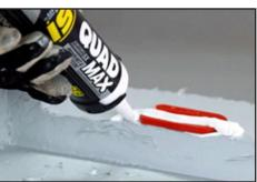
9 Apply a continuous 3/8" rounded bead of OSI® QUAD® Max to the head and side buck edges of the window flange.
