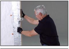
**9** Apply the head flashing tightly to the wall sheathing, extending it at least 1" past the flashing tape for the side jambs. Use the J-roller to remove any air pockets.
