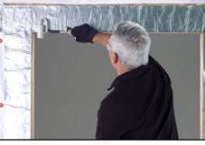
**10** Apply a fillet bead to the backside where the brickmould meets the jamb and back seal all miter corners with a bead of OSI® QUAD® Max. Then apply a 3/8" bead of OSI® QUAD® Max to the outer edge of the brickmould.
