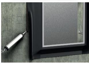
Apply strands of TEROSON AD KDS FR to the substrate using either a manual or a compressed air gun (pressure 0.5 to 5 bars). Afterwards, press the sealing strip into the adhesive paste while it is still fresh and skin-free. Roll the strip over with a pressure roller. On very uneven substrates, TEROSON AD KDS FR can be used to fix the upper edge of the TEROSON FO 2 FR sealing strip and to seal it against water penetrating from behind.
