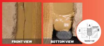
• Dimension C beyond standard maximum depth. This will debilitate joint movement capability causing fissures and fractures • Slow cure due to excessive sealant depth may compromise sealant performance • Dimension B beyond standard maximum depth
