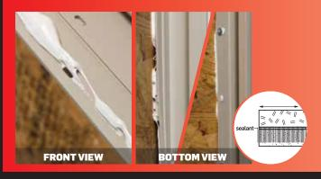
Substrate movement will smear the sealant breaking down the capacity to maintain a gasket seal. This will leave insufficient amount of sealant to accommodate joint movement allowing for air and moisture infiltration For more information, references and supporting technical documents call OSI Technical Customer Service at 800-624-7767 and visit **OSITough.com**
