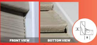
• Dimension A under 1/4" minimum. This will compromise the sealants adhesion performance and ability to sustain joint movement capability • Reduced sealant volume will diminish sealants ability to accommodate joint movement
