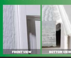
A control joint is formed when two similar or dissimilar materials meet or when substrates do not form a right angle. This joint will require both a backer rod and sealant for proper application.
