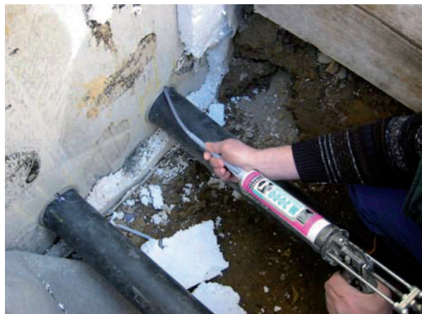
Fig. 4 Injection of the Tangit M 3000 Expansion Resin.
