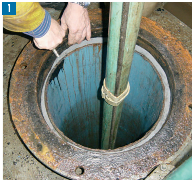
Insertion of the Tangit sealing hose
