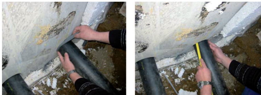
Fig. 2 Insertion of the Tangit M 4082 sealing hose
