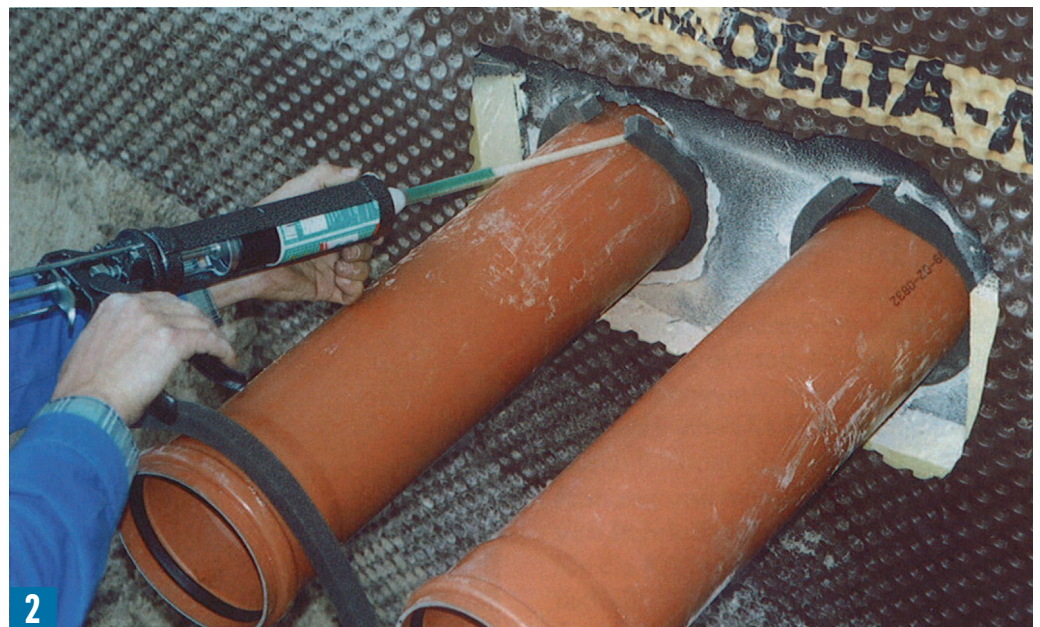
Filling of the cavities on the outside.
