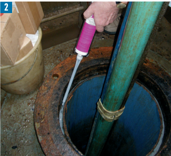
Injection of the expansion resin into the joint
