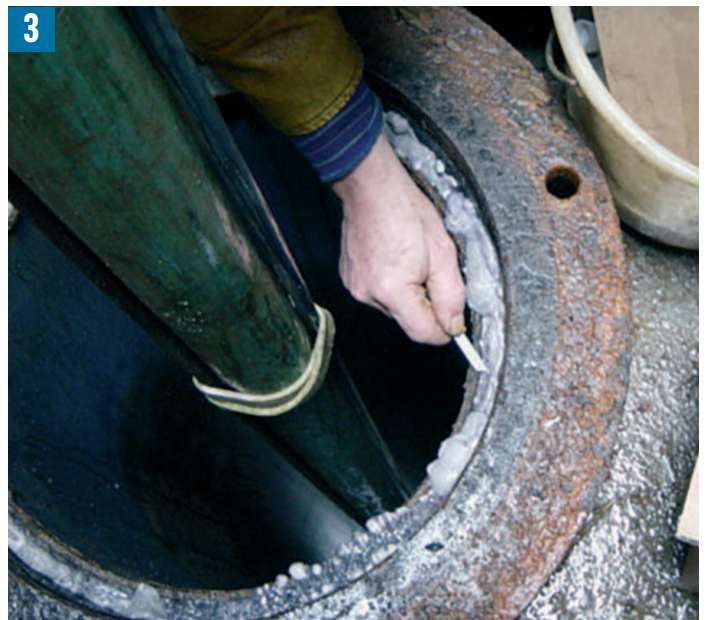
Excess cured Tangit M 3000 is trimmed off.
