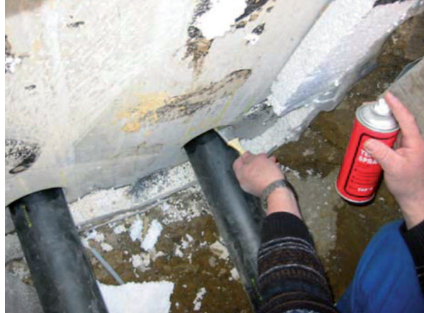
Fig. 3 Coating of the PCP pipes with Teflon
