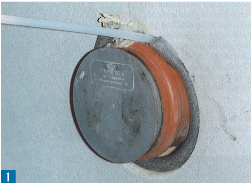
Filling of the cavities on the inside.
