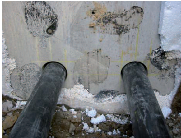
Fig. 1 PCP district heating pipes in the trench
