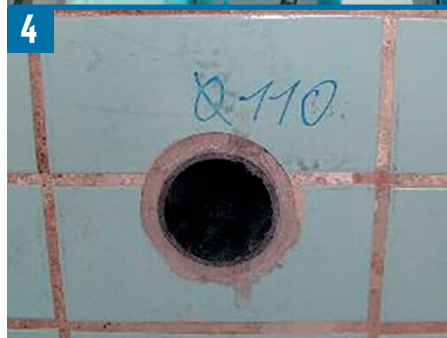
4 Finished state of the installed Tangit system
