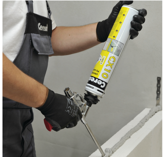
Foam application during joining of aerated concrete blocks
