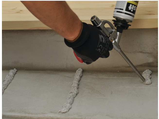
Foam application for mounting stairs
