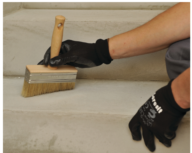
Cleaning the substrate
