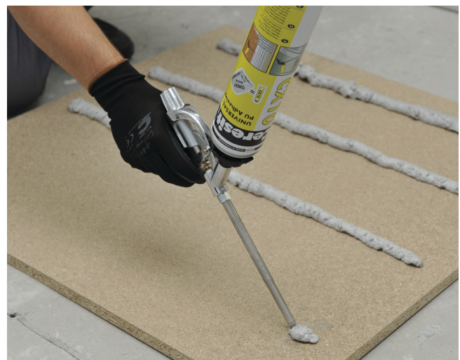
Foam application on the board
