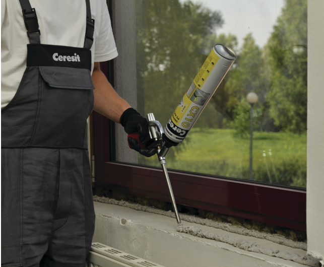
Foam application for window sill installation
