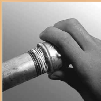
Ideal connection between plastic and metal. Easily re-adjustable to ensure a snug fit, e.g. of a tapping or feeder point.
