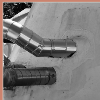
Mortar bulkhead around a metal pipe passage.
