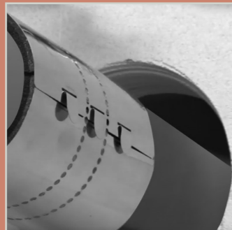
Before inserting the sleeve, carefully thread in all straps and completely turn them back.
