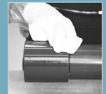
Cleaning and activation of the bonded surfaces is absolutely essential to ensure a reliable bond.
