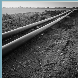
Installation of a sewage pipe in civil engineering.
