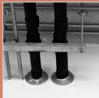
Core product for the classical mortar bulkhead. FP 300 can be applied by hand or mortar pump.
