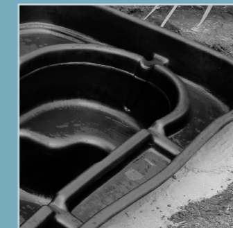
Solvent welding of PVC sheeting, e.g. for installing ponds and swimming
