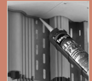
FP440 fills joints between the panels used for cladding the penetration of a ceiling.
