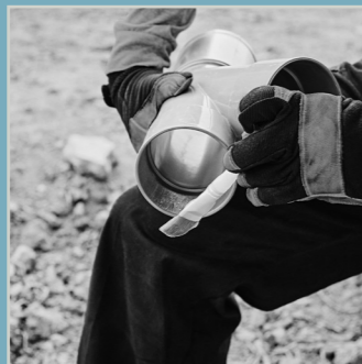
The pipe adhesive can be applied with a soft paint brush.
