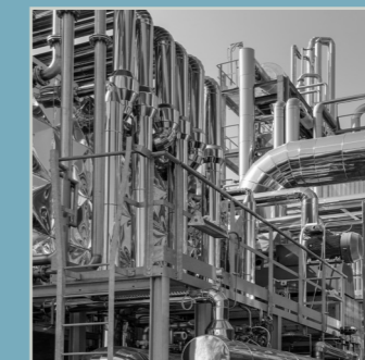
Construction of chemical and metal processing plants.
