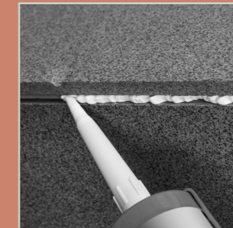
On ceilings FP 440 provides a connection between the paneling and the building structure.
