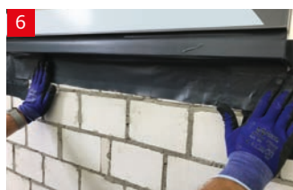
Molding the sealing strip to the surface
