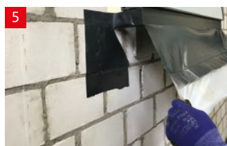
Easy removal of the protective film
