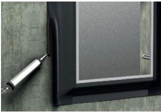
Apply strands of TEROSON AD KDS to the substrate using either a manual or a compressed air gun (pressure 0.5 to 5 bars).
