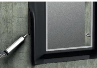
Apply strands of TEROSON AD KDS to the substrate using either a manual or a compressed air gun (pressure 0.5 to 5 bars). Afterwards, press the sealing strip into the adhesive paste while it is still fresh and skin-free. Roll the strip over with a pressure roller. On very uneven substrates, TEROSON AD KDS can be used to fix the upper edge of the TEROSON FO 3 sealing strip and to seal it against water penetrating from behind.
