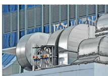
HVAC Air Compressor Pumps
