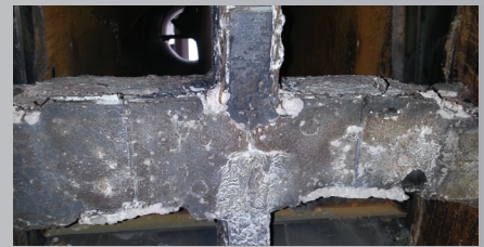
PC 7000™ coated burner tip after 1 full year of service life. (50% of coating still remaining)
