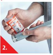
Wind onto one of the first pitches of the thread and continue in random cross pattern around the thread.
