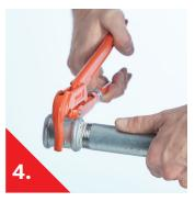
Screw on and fasten the joint with a pipe wrench. Reposition if necessary.
