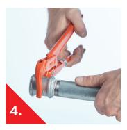
Screw on and fasten the joint with a pipe wrench. Reposition if necessary.
