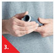
Cut the LOCTITE 55 sealing cord with the incorporated cutting device and press the loose end of the thread.
