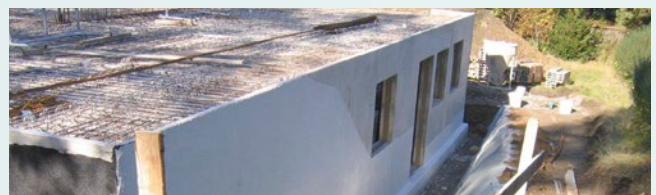
Basements and foundations
