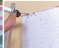
Filling in gap between boards.
