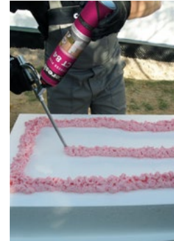
Fixing EPS board in thermal insulation system.
