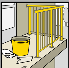
Fixing balcony railings
