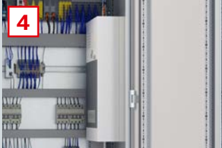
Cooling device for switch cabinet temperature control
