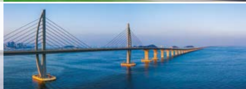
Project: HK-Zhuhai-Macau Bridge Category: Wall & Floor Location: Hong Kong
