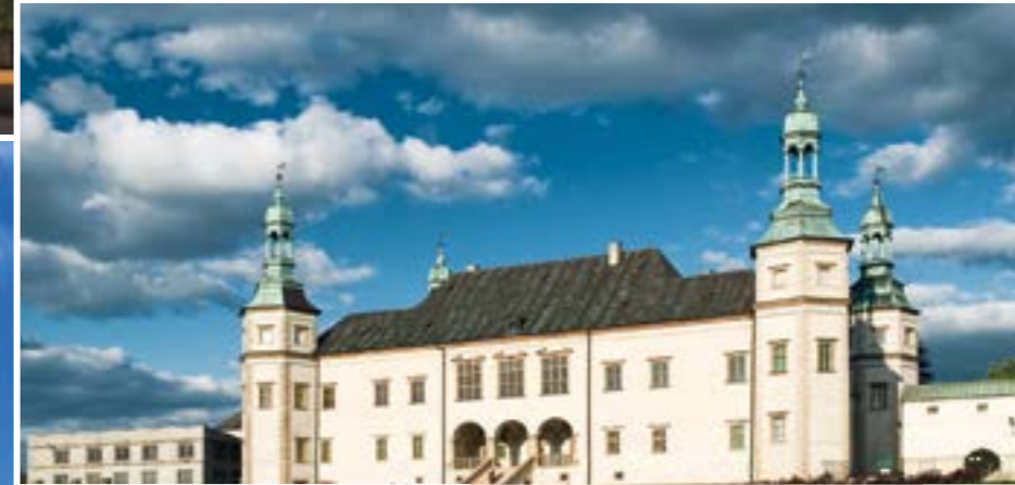
Project: Kielce National Museum Category: Facade Location: Poland
