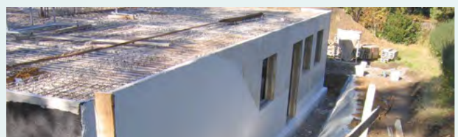
Basements and foundations
