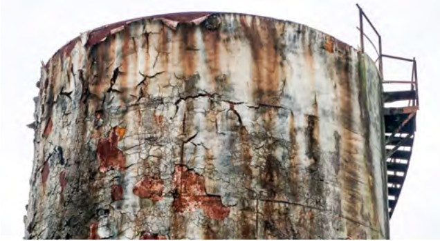
Without concrete protection
